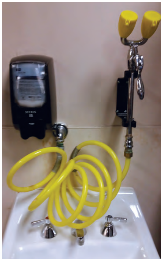
Figure III.1. OSHA regulations require facilities to provide an eye wash station and an emergency shower wherever employees are exposed to chemicals. The stations must be checked regularly to ensure that they are functioning properly.
